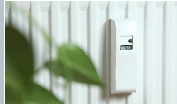
Heat Cost Allocator
