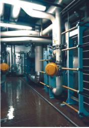
Water plays a critical role in the manufacture of semiconductor products and because of the extreme sensitivity of processes, only ultra-pure water can be used. This is created by reverse osmosis and de-ionization.
